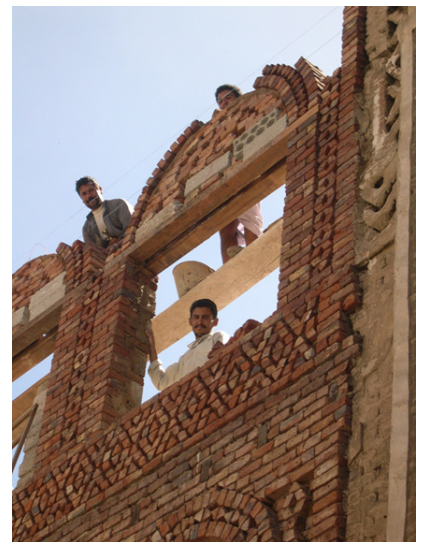
Figure 4: Brick arches and detailing applied as veneer on a concrete block wall.
